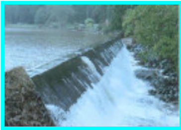
Eastwood Lake Dam, Chapel Hill, NC
